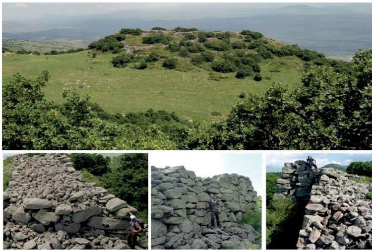
Рис. 1. Teghenik fortress, Cyclopean walls (photos of the author)
